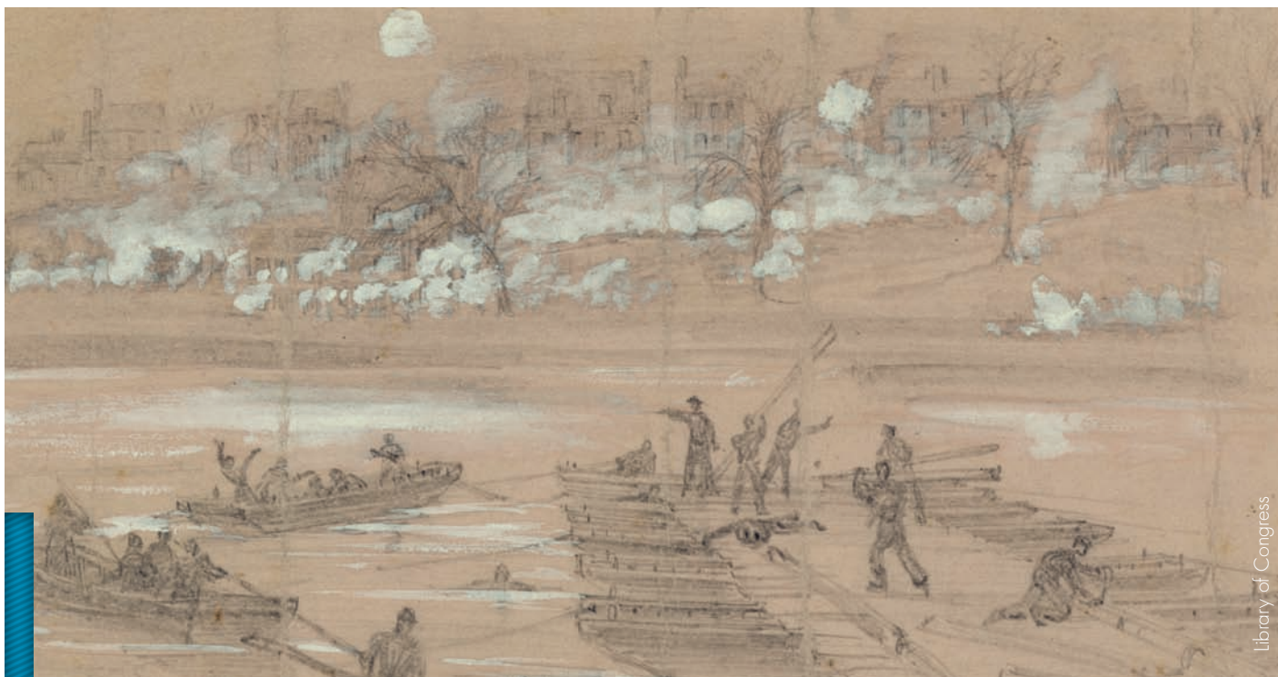
Union Army engineers build a pontoon bridge across the Rappahannock River into Fredericksburg, 11 December 1862, drawing by Alfred R. Waud
