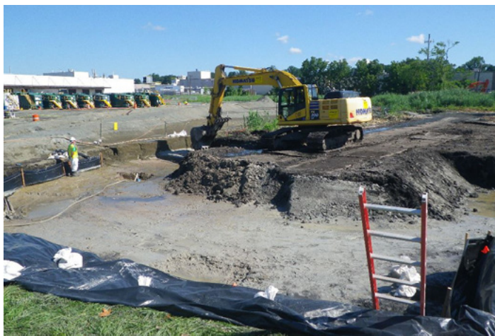
Remedial excavations of a wetland on a commercial property in Maywood, New Jersey. Water management was a challenge, as evidenced by the row of portable water storage tanks in the background.
