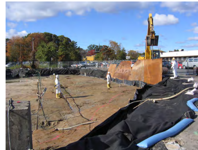
Radiation technicians provide support during the removal of sheet pile used at this Maywood, N.J., vicinity property.
