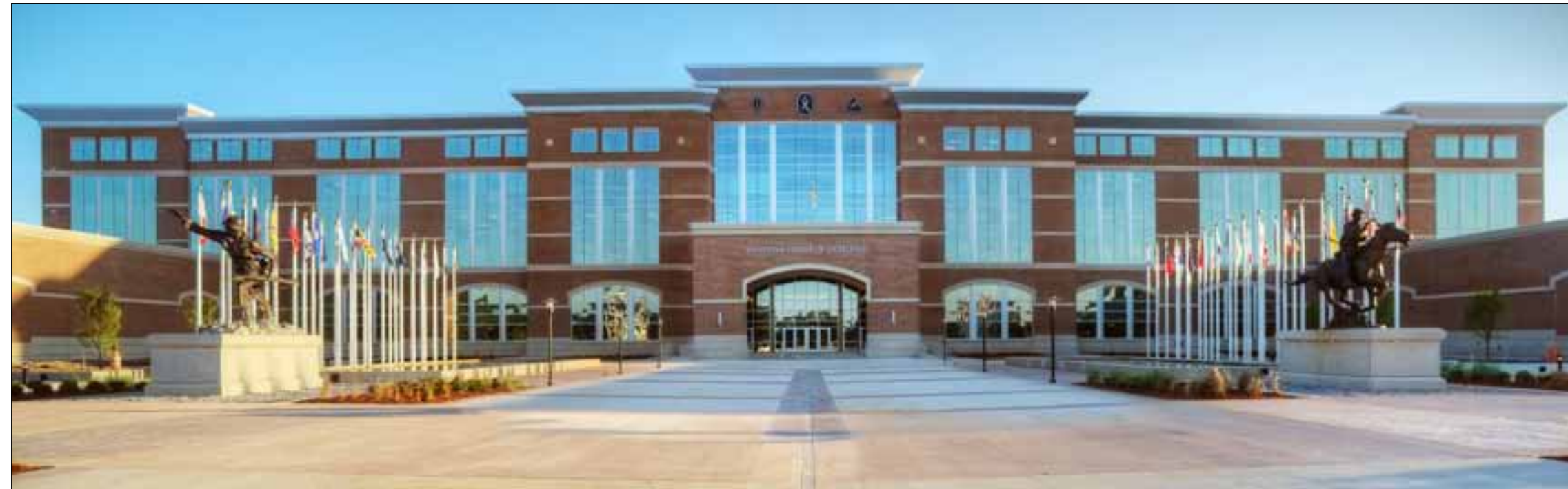
The U.S. Army Corps of Engineers Savannah District managed and executed the largest renovation project ($168 million) in the Army, the Maneuver Center of Excellence Headquarters at Fort Benning, Ga. The facility was named after two Medal of Honor recipients, Spc. Ross McGinnis and Cpl. Jerry Wickam, during a dedication ceremony Sept. 23, 2011. Construction began in late-2008 and was performed by prime contractor McCarty Corp. (Photo by Kristian Ogden)
