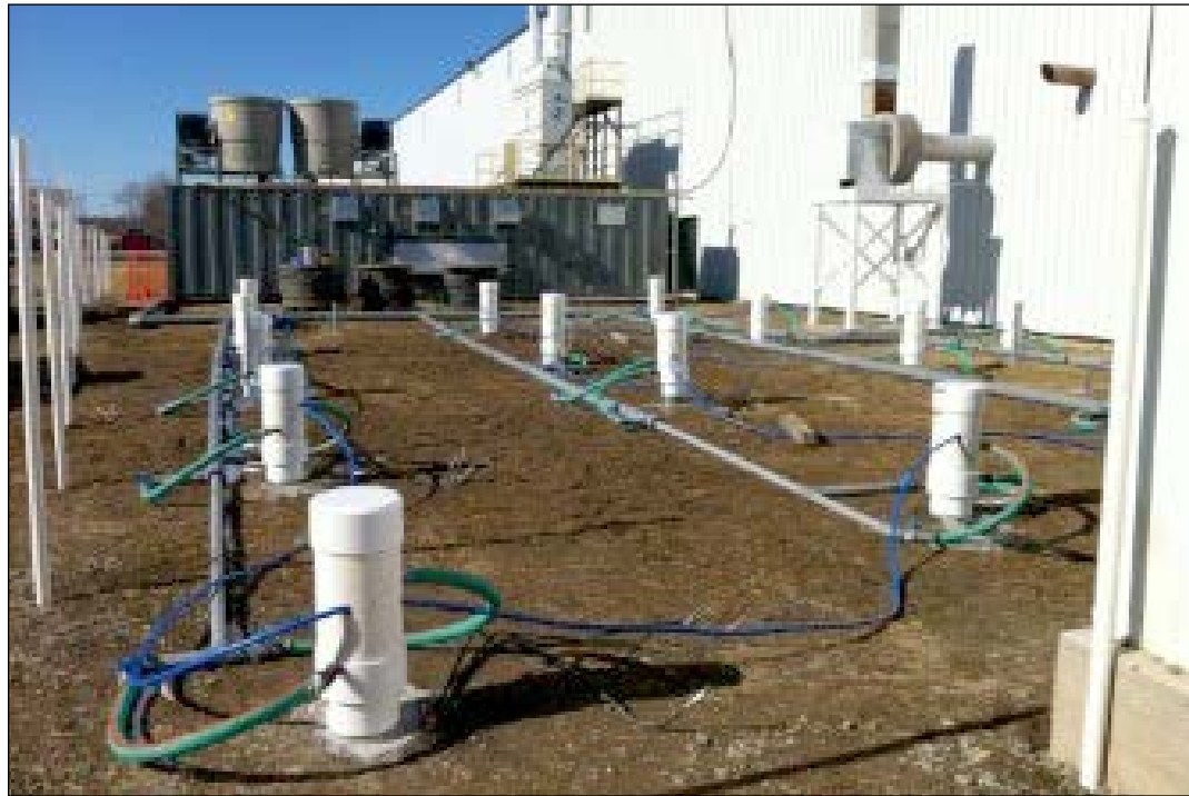
During the electrical resistance heating process, electrodes deliver power to the subsurface to lift contaminants out of the soil. This environmental remediation method works in all soil types and can be applied under operating facilities and public areas.
