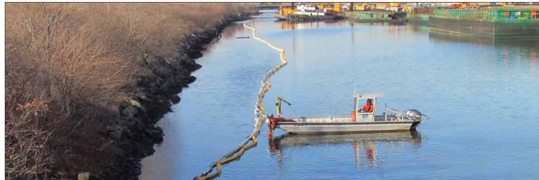
A worker installs oil booms at Indiana Harbor and Canal, Nov. 27. (Photo by Vanessa Villarreal)
