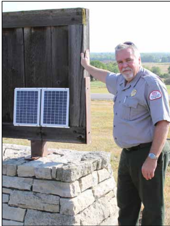
Jim Franz, natural resource manager for Melvern Lake in Melvern, Kan., shows off a solar panel installed to provide energy for LED lights that light the large entrance sign to the lake. (Photo by Diana McCoy)
