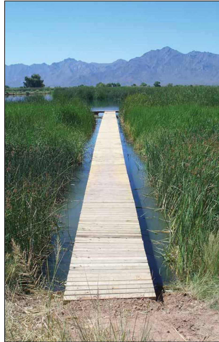
The Tres Rios Environmental Restoration Project, Phase II Flow Regulating and Overbank Wetlands, Salt River, Ariz. earned the Chief of Engineers Award of Excellence in the Environmental Category. (Courtesy photo)
