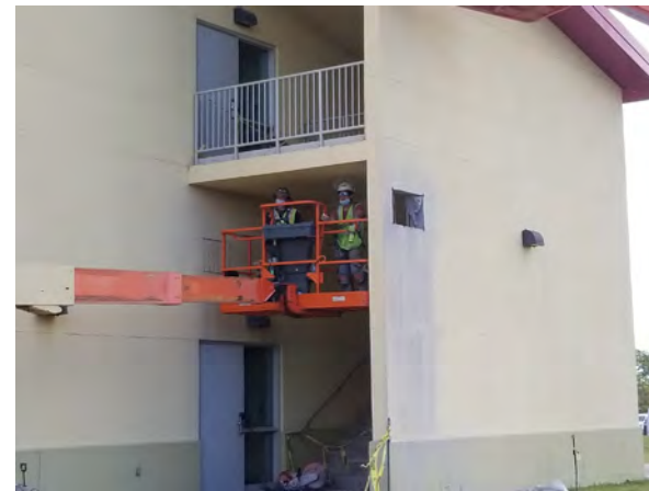
Supply Duct Cutoffs for DOAS HVAC System.
