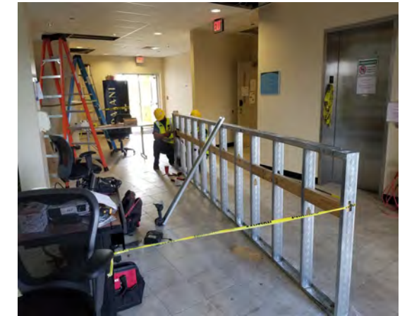
Nurses' Station Installation in Progress.
