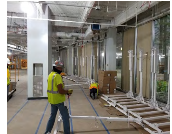
29APR20: 1 st Floor Bed Lighting Assembly and Storage
