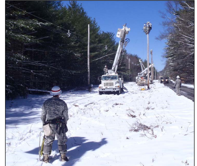
Restoring distribution line service
