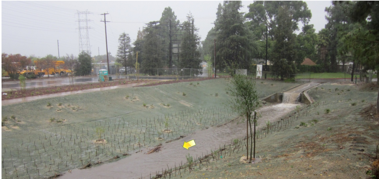
Figure 1: Atwater Park - 'daylighted' storm drain, just after construction, Nov. 2011
