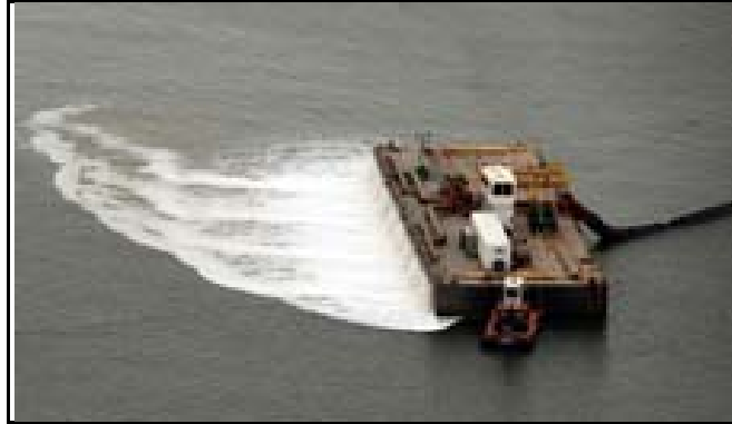
Figure 2.2-4. Spill barge designed for the Craney Island project.
