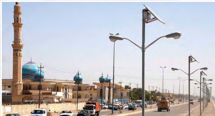
Solar-powered lights will guide traffic at night on a street in front of a mosque in Fallujah, Iraq. The Corps is installing solar-powered lighting as part of infrastructure reconstruction work in Iraq.
