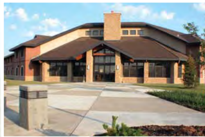
The Lodging Facility, Niagara Falls Air Reserve Station, N.Y., offers water efficiency, energy saving features and is built using a percentage of recycled materials.
