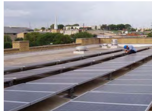
A worker installs photovoltaic solar panels on Bldg. 1350 at Fort Sam Houston, Texas.
