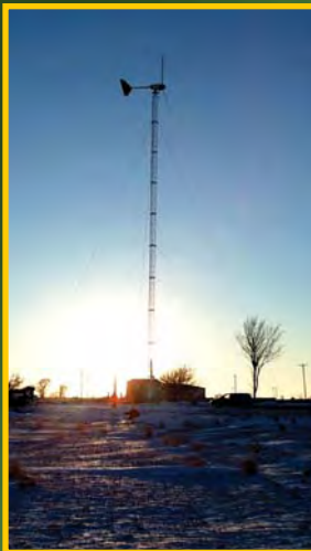
The wind-powered turbine at the Nebraska Ordnance Plant, Mead, Neb., supplies approximately 30 percent of the power needed for a groundwater recirculation well. The treated water is also beneficially used to irrigate crops.
