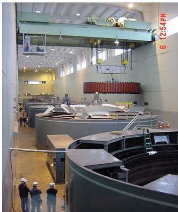
Cab-Operated Class I Overhead Crane
