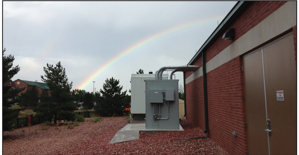
A back up power diesel generator is integrated into a microgrid power system at Fort Carson, Colorado. (U.S. Army photo)
