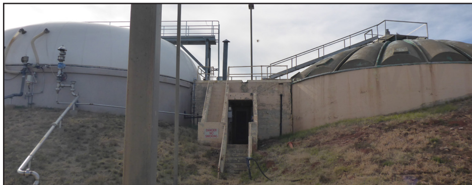
Anaerobic digesters at the Fort Huachuca, Arizona, Waste Water Treatment Plant have the ability to help reduce the carbon footprint of waste on an installation and help it meet Net Zero Energy goals. (U.S. Army photo)
