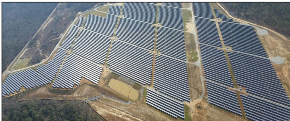
At Fort Benning, Georgia, 133,950 solar panels make up the 30-megawatt solar array. It's just one of the U.S. Army renewable energy projects that total close to 125 megawatts of power in Georgia and Alabama. (U.S. Army photo)
