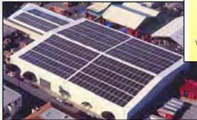
Renewable Power Production
