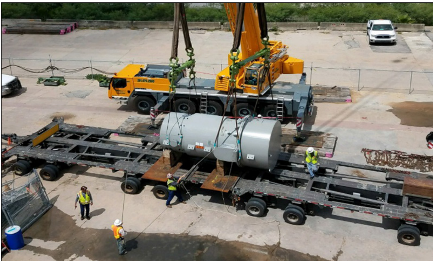
The reactor pressure vessel from the STURGIS is carefully loaded onto a transport vehicle inside a specially designed shielded shipping container.
