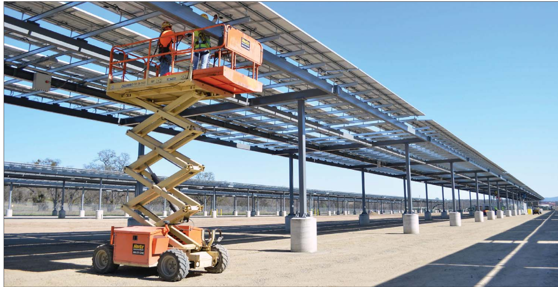
Construction workers complete electrical connections on phase two of a solar microgrid project at Fort Hunter Liggett, Calif. Sacramento District managed construction of the project, awarding contracts of $8.4 million for phase one and $9.7 million for phase two. (Photo by John Prettyman)
