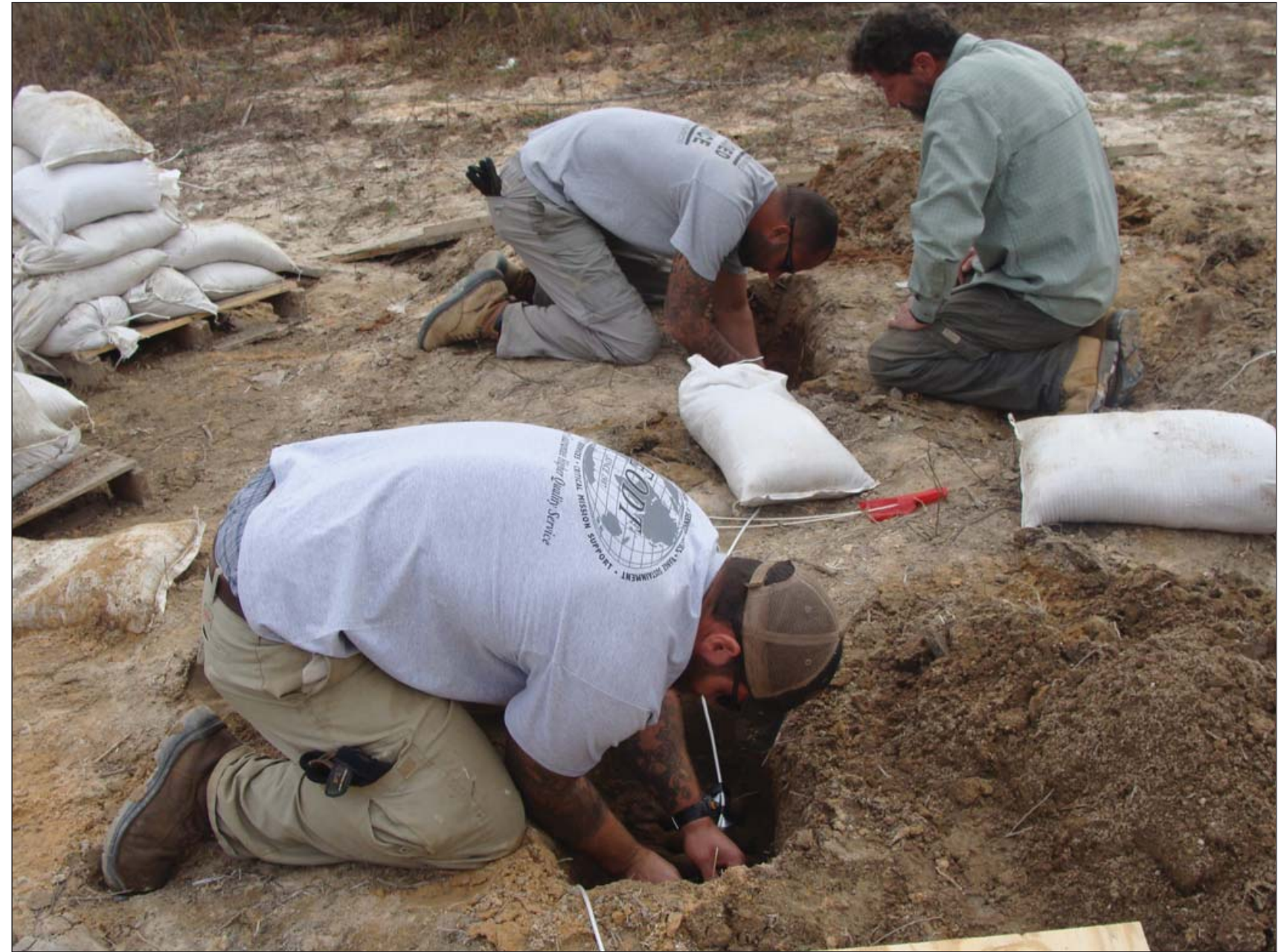
Workers install wiring to detonate unexploded munitions discovered at the power corridor site on former Camp Wheeler. (USACE photo)
