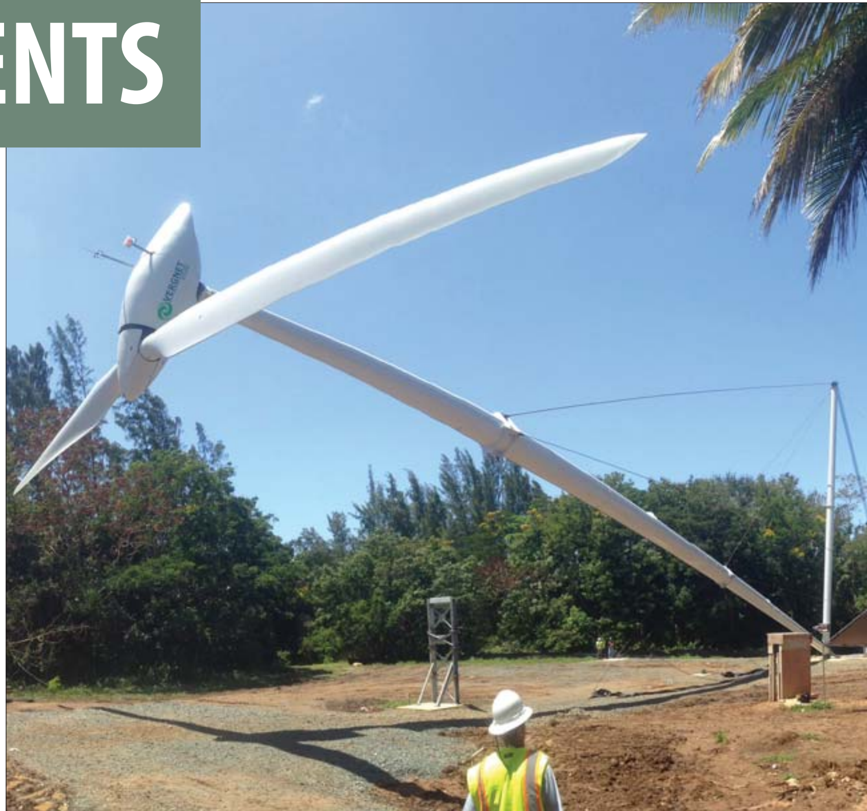
The first of three 275 kilowatt wind turbines is erected April 18 on Fort Buchanan, Puerto Rico. The turbines are part of a large, multi-project renewable energy/energy reduction and Net Zero Water effort. The U.S. Army Engineering and Support Center, Huntsville, awarded a $34 million task order contract to Johnson Controls Government Systems, Milwaukee Wis., on Dec. 22, 2012, to install wind power generation, solar photovoltaic systems, water conservation measures, and other energy conservation measures at Fort Buchanan. (Photo by José L. López)
