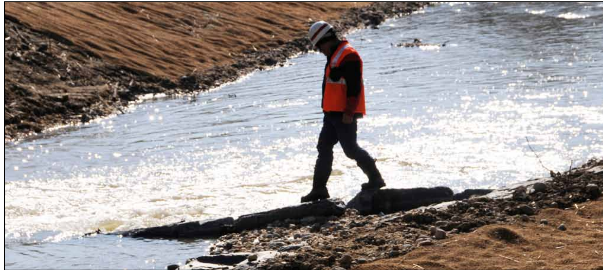
Ben Soleimani, district hydraulic engineer, inspects the Paint Branch project. (Photo by Andrea Takash)
