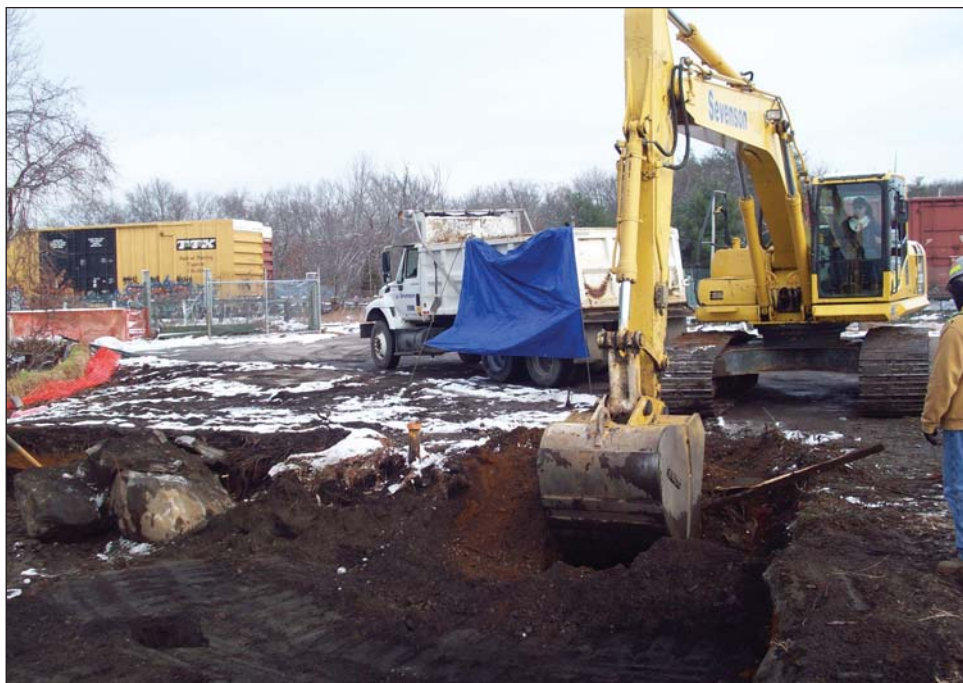
A contractor works at the Hatheway & Patterson Superfund Site. (Courtesy photo)
