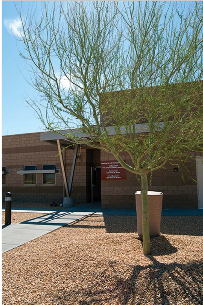
The 11th Armored Cavalry Regiment’s new Company Operations Facility at Fort Irwin, Calif., is designed to use less energy for heating and cooling. (Photo courtesy of RQ Construction)
