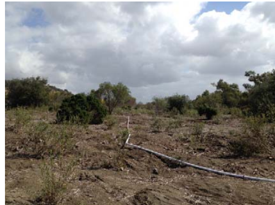
Figure 3.3-10. Irrigation line hose connections and shut-off ball valves in several locations
