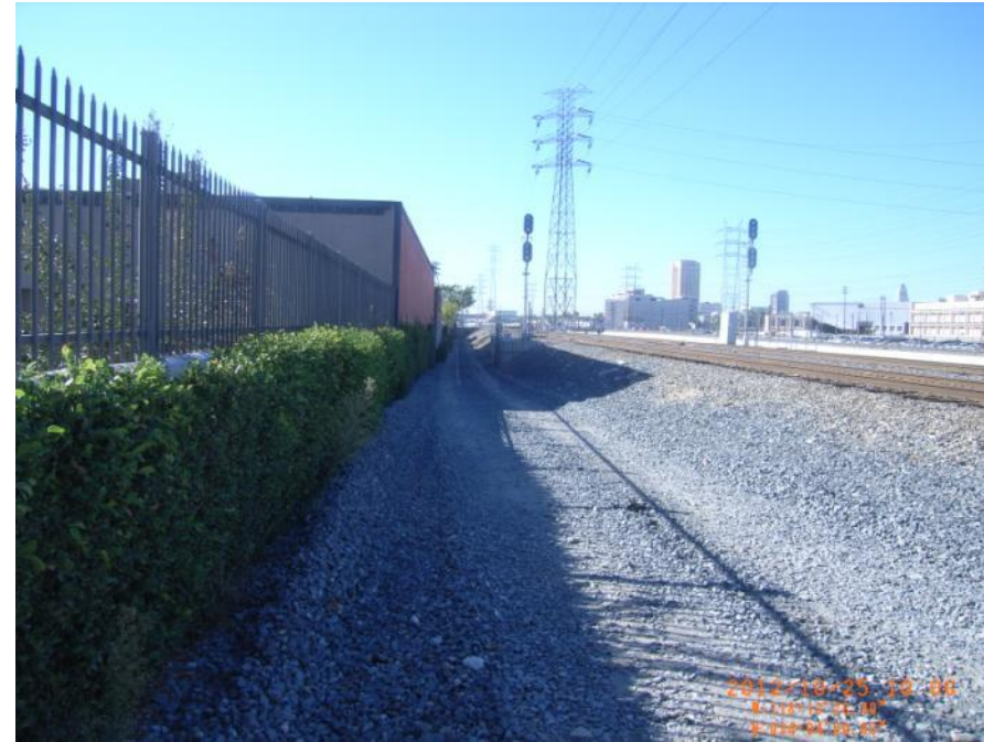
Photo 3: View looking downstream at N. Main Street. LAR 5 on right side. Not a levee condition. Ground in immediate foreground at approximately the same elevation of the wall depicted in Photo 2.
