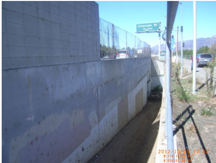
Photo 7: Equestrian ramp and tunnel entrance. Note crest on right, highway on left. Tunnel and culvert at base of down-ramp in center.
