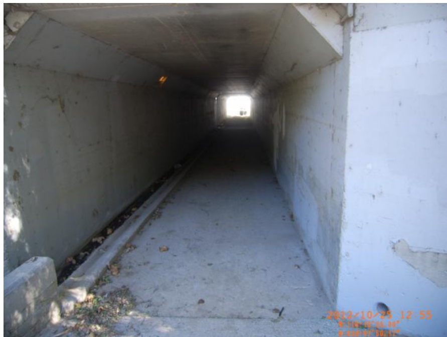
Photo 8: Landside of tunnel culvert at end of tunnel in background. Tunnel height allows horse and rider to pass through without rider bending over. Note small wall in foreground as it is the same wall depicted in Photo 9.
