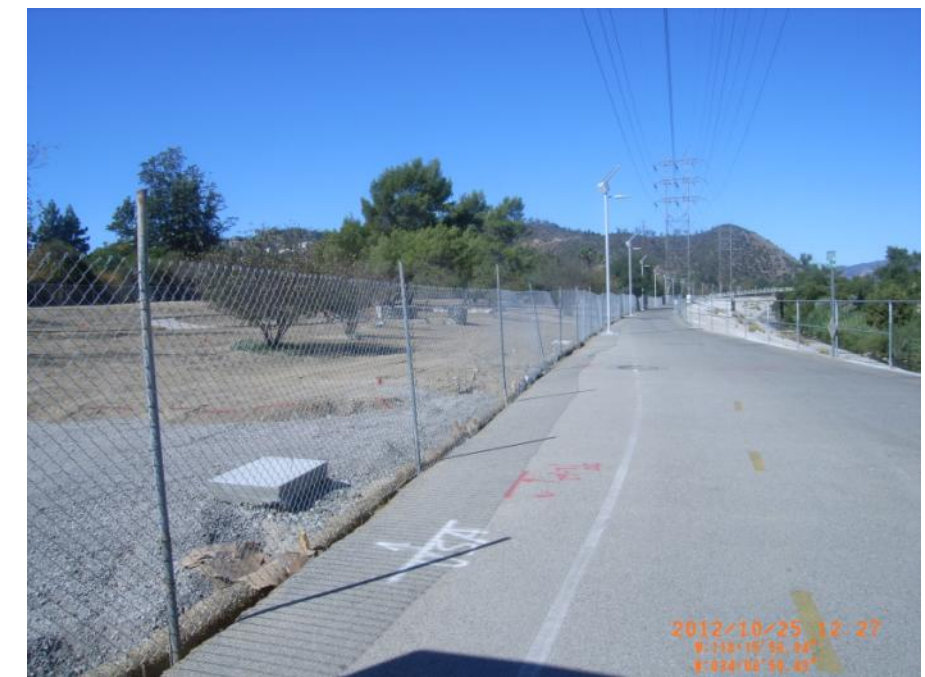
Photo 6: Looking upstream along LAR 3 just upstream of Hyperion Ave. Not a levee condition. Grades for park are above crest.
