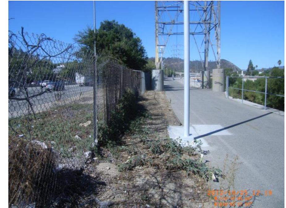
Photo 5: On crest of LAR 3 looking upstream. Not a levee condition. Although landside is slightly lower than crest. Flow would be directed along I-5 (on left) and the crest of the highway is above the crest of LAR 3.
