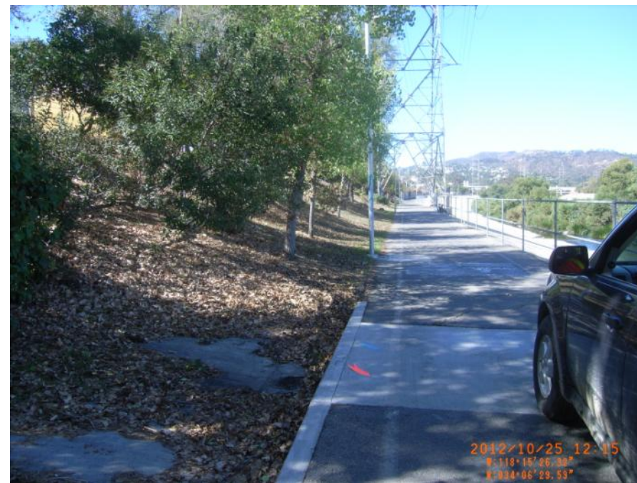
Photo 4: Looking upstream near downstream end of LAR 3. Not a levee condition. Ascending slope to high ground on landside. Vegetation would be within the VFZ if this portion is to remain listed as levee or is required for levee support upstream or downstream.
