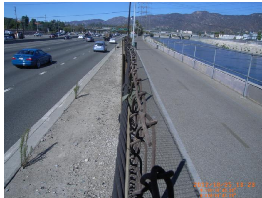
Photo 10: Looking upstream on LAR 3 near Gene Autry Museum. Levee condition of approximately 2 to 4-feet exists and flow would be directed on I-5 and along levee. Southbound lanes are higher than northbound lanes.
