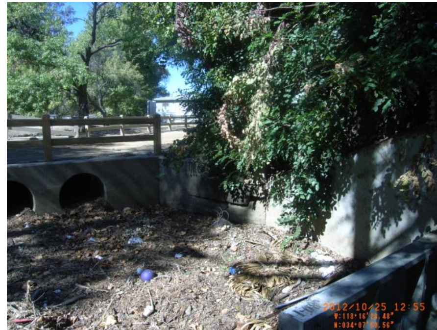
Photo 9: Landside of tunnel looking upstream. Wall in foreground is the wall depicted in Photo 8. The building in background is at approximately same grade as top of tunnel.
