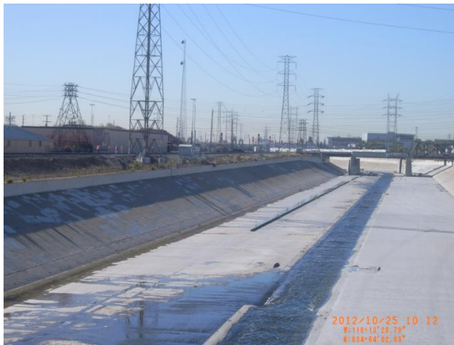
Photo 2: View looking downstream at N. Main Street. LAR 5 on left side. Not a levee condition. Railroad embankment with ascending slope above top of wall. Photo 3 depicts landside condition further.
