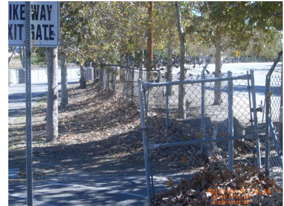
Photo 11: At Ferraro Fields looking downstream on LAR 3. Levee condition beyond right of photo and vegetation on landside crest.
