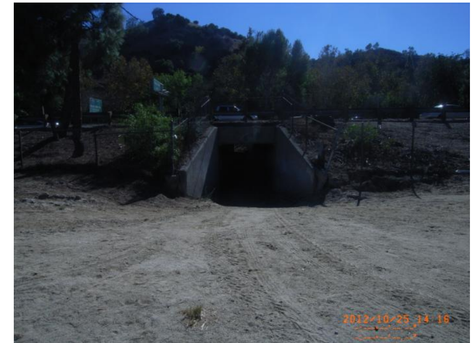
Photo 12: Equestrian undercrossing on landside of LAR 3. Photo taken at landside crest.
